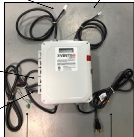
Meridian Control Panel
